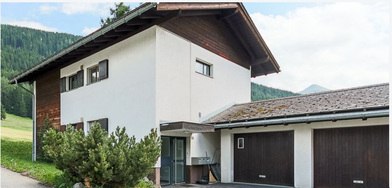
Building from outside
